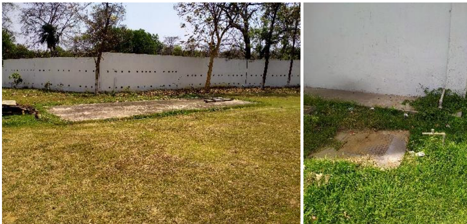
Rainwater Harvesting Pits
