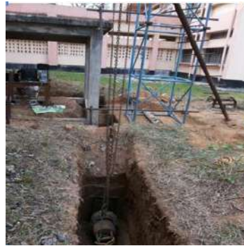
Construction of trench
