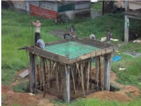
Construction of roof
