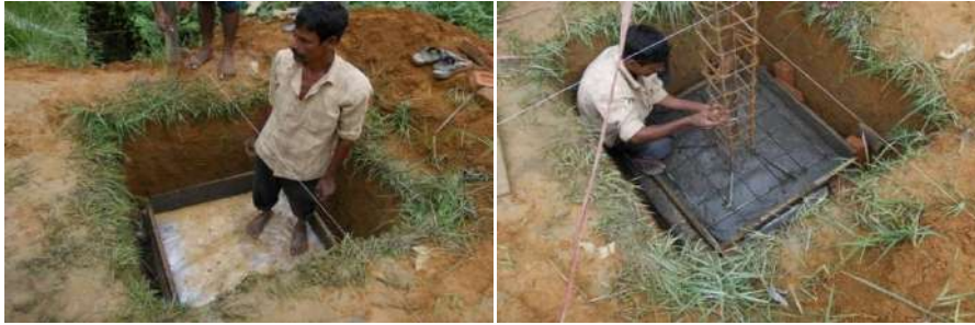
Construction of foundation
