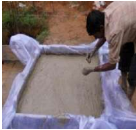
Figure 4. Construction of footing over the clay damper is shown in figure 5
