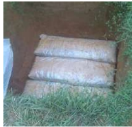
Figure 4. Construction of footing over the clay damper is shown in figure 5
